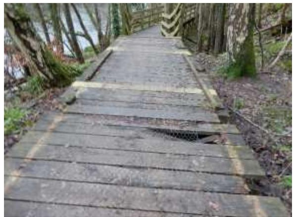
Between Mauldslee Bridge and Cardie's Bridge on the B701 there are numerous wooden footbridges, some only 90-100 cm wide, and some with rotten planks.
