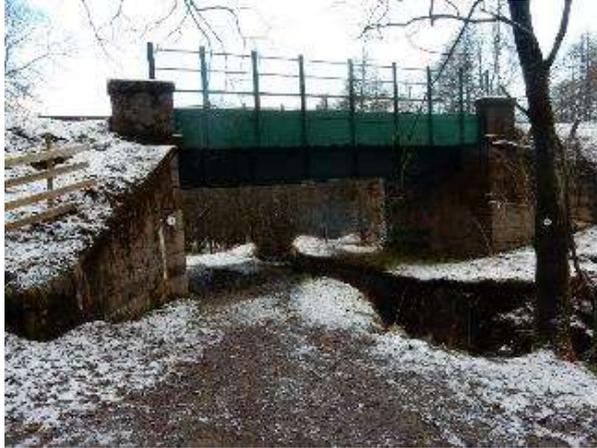
The path north of the railway has recently been upgraded – please take particular care to avoid damaging the lovely new surface. At OSGR NS259967 there is a 90 cm wide wooden footbridge over the burn. At the time of survey, some of the decking appeared rotten, and the weldmesh reinforcement laid on top could present a hazard. The route managers are investigating replacement.
